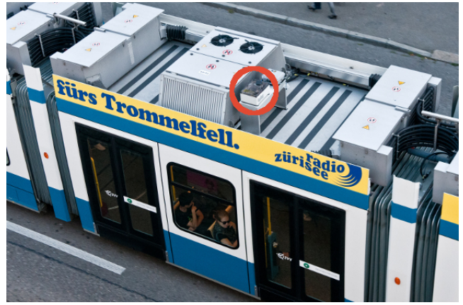
Figure 11: Air quality sensor node installed on top of a streetcar of the local public transport network.
